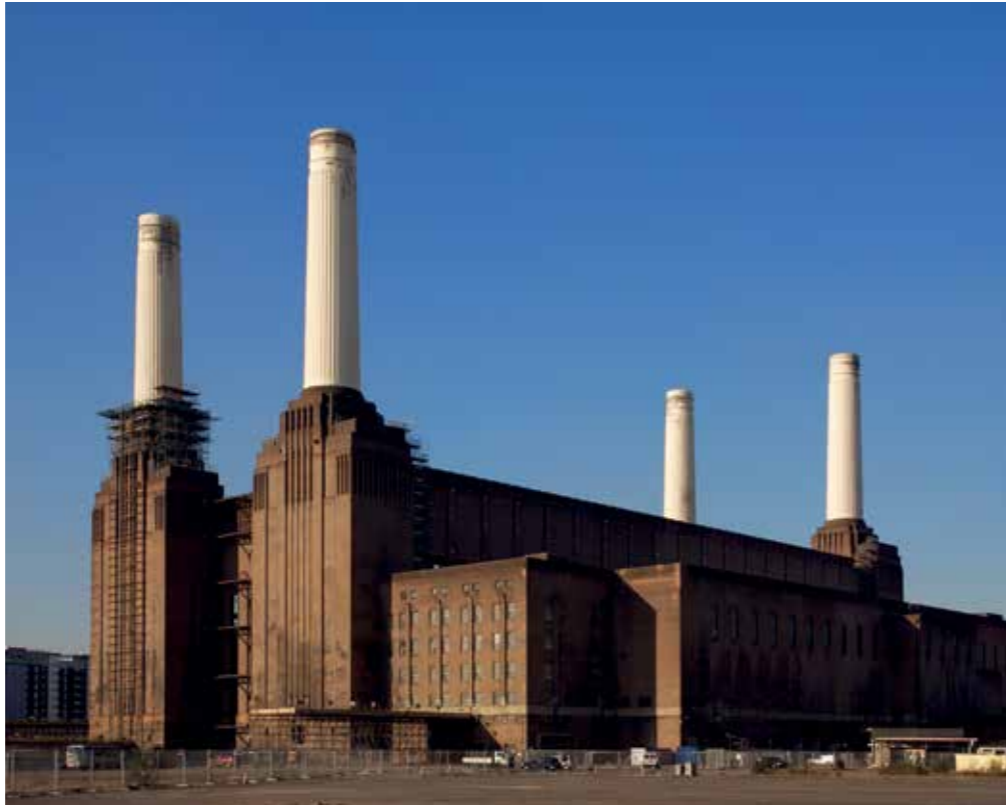
The Power Station in its current form
